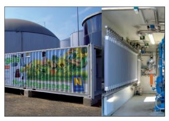
**Figure 3:** View of the shipping container used for the membrane up-grading equipment (left) and the membranes themselves inside the container (left side of right photo).
